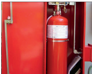
Integral dry chemical fire suppression
