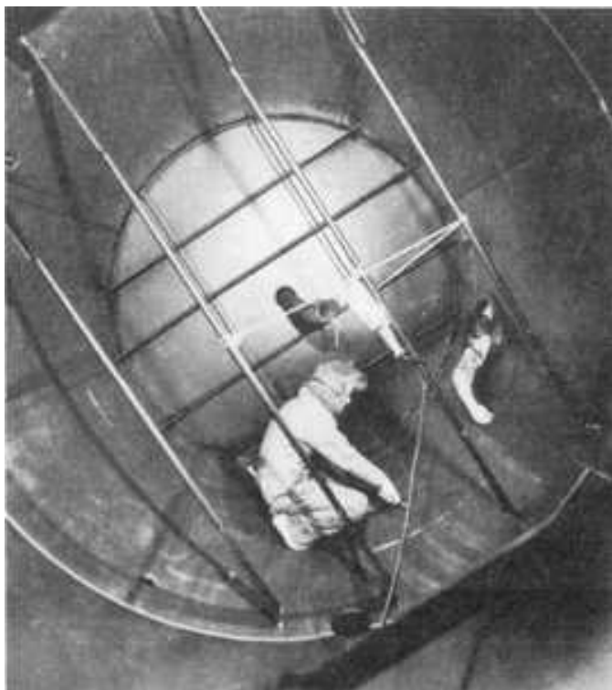
Inside a tank being lined, the area is being rolled with a rubber roller to eliminate all air trapped between the sheet and the metal surface.
